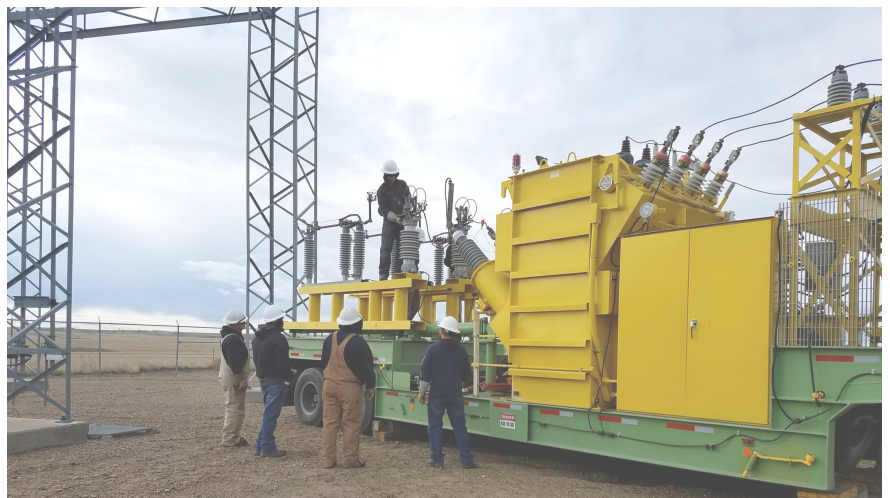
Above: Hill County Electric Crews work with NorVal Crews to stabilize the mobile substation.
