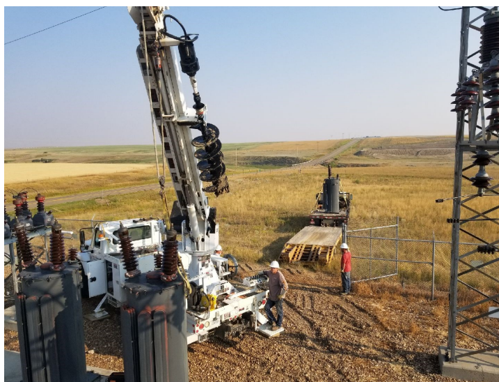
During the Electro-Test transformer testing they discover a transformer that needs to be replaced in the Benrud Sub. The crews install a temporary transformer until a permanent one arrives.
