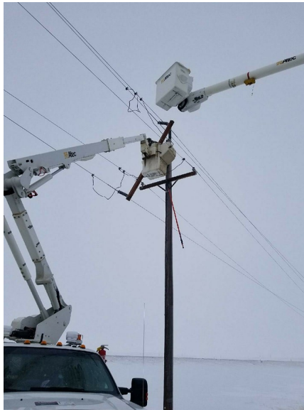
Crews repair a broken cross arm.
