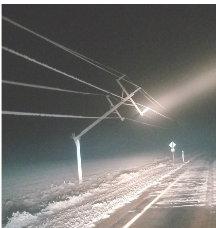
Left: a broken pole is visible with the spotlight. Right: the Opheim Sub encased in an icy mix of frost.
