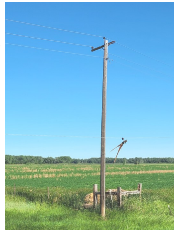
A broken cross arm was found West of Glasgow after the storm.
